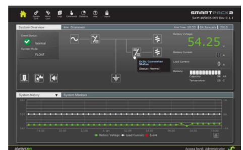
Status of DC/DC converters in Smartpack2 web
